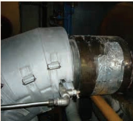
Touch temperature was reduced from 85°C (185°F) with ceramic fiber ...
