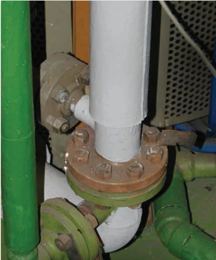
LEFT: Operators work continuously in the web of pipes, often coming into contact with them. Aerogel insulation reduced the touch temperature to safe levels, reducing the risk of injuries.
