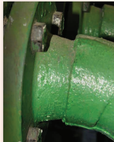
ABOVE: The Pyrogel® insulation was easily painted — gray for gas, green for hot water — to identify the fluid in the piping.
